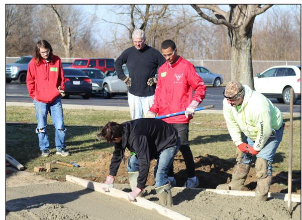
Chillicothe High School students taking a Construction Craft Laborer course poured concrete to repair an area of walkway near the superintendent's office that had been damaged by a sinkhole.
